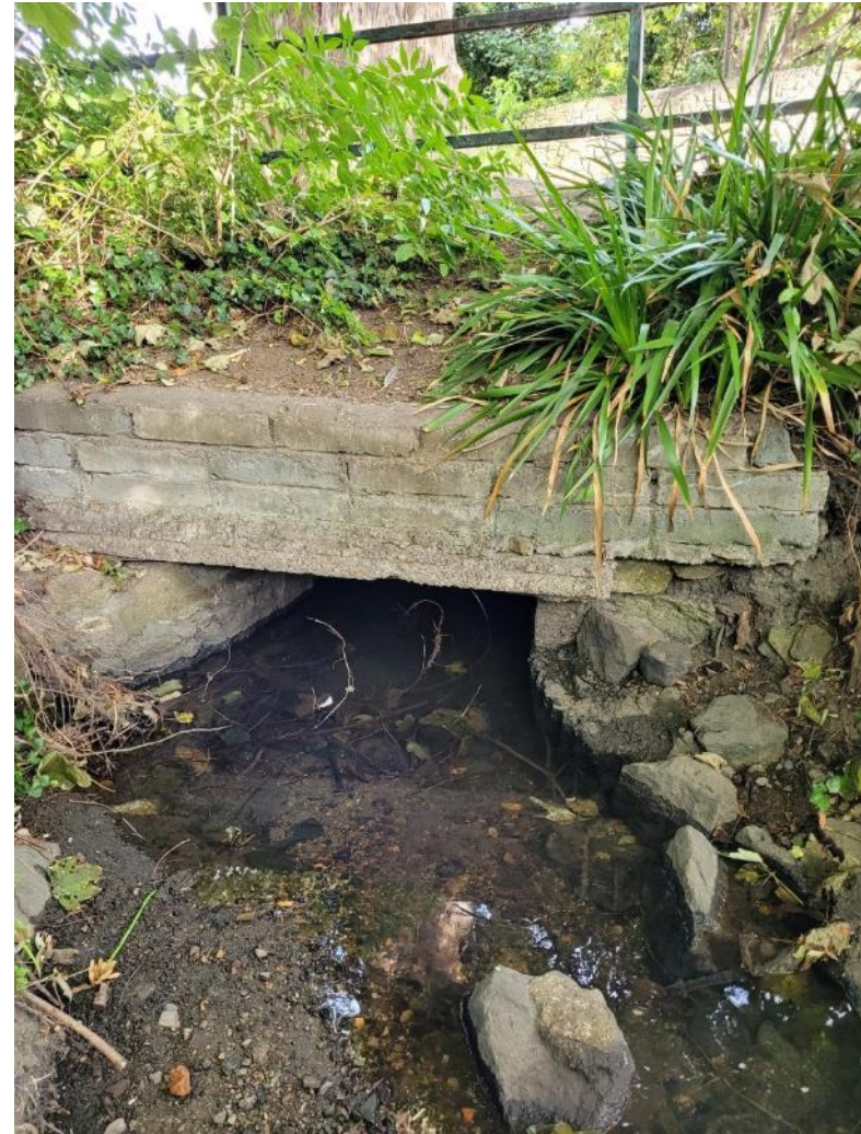
Figure F Site 2 - Facing downstream
