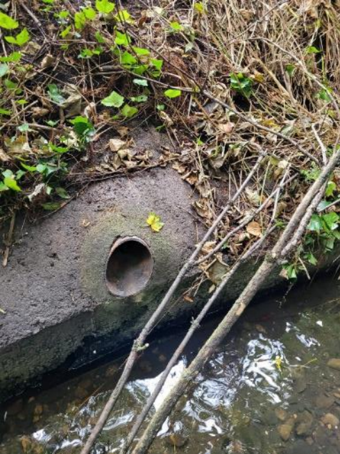
Figure D Site 1 - Storm drain
